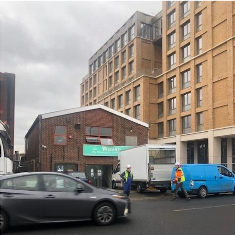
View of the existing principal elevation
